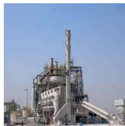
The CCM plant in Madinah Industrial City
