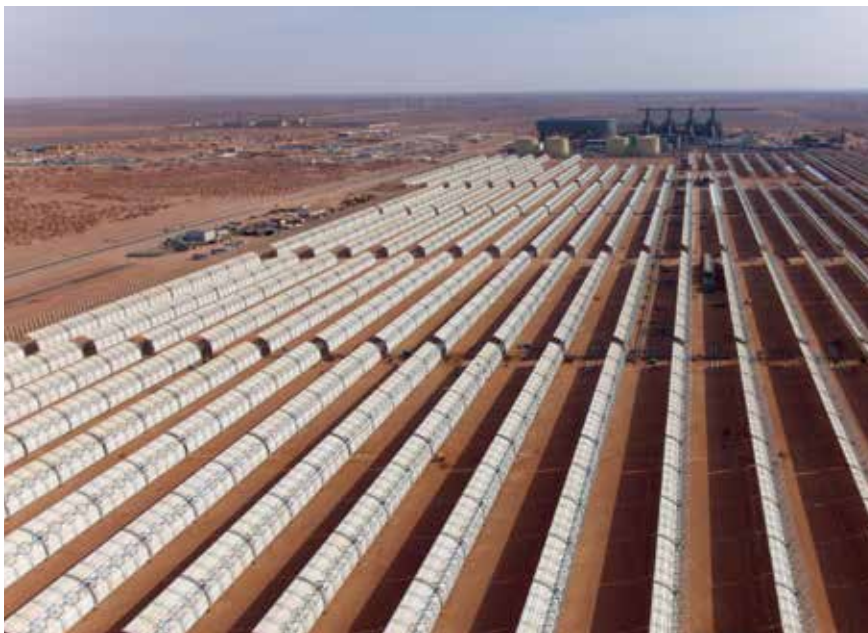
The integrated solar combined cycle (ISCC) power plant uses a combination of solar power and natural gas to fuel our Wa'ad Al-Shamal plants, contributing to the national goal of increasing the share of renewable energy in the power mix.
