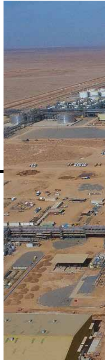
Above Our phosphate complex in Wa'ad Al Shamal includes a beneficiation plant and phosphoric and sulfuric acid plants
